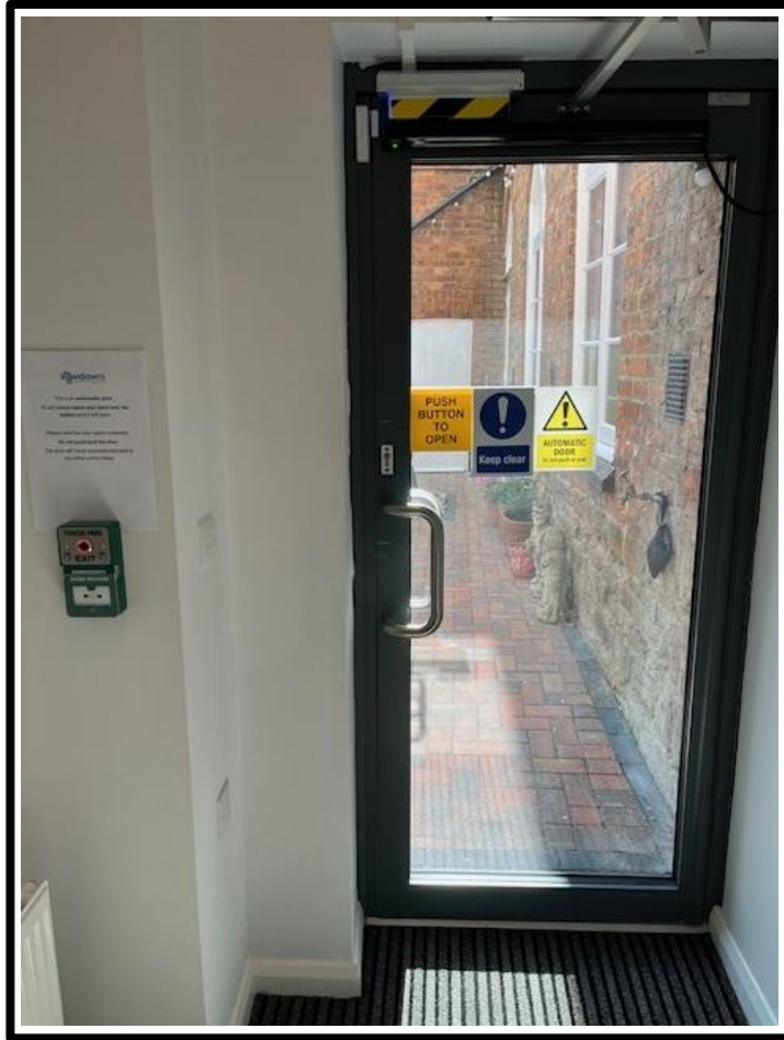
1. Ground floor internal, garden exit.
