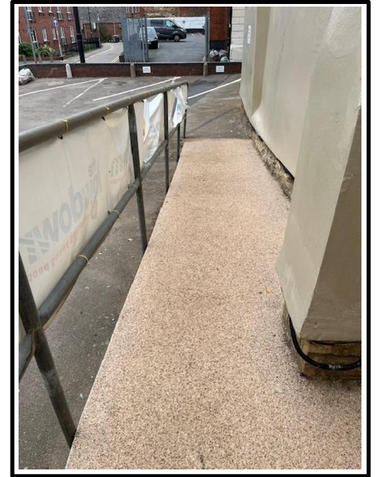
3. Accessible ramp to car park.
