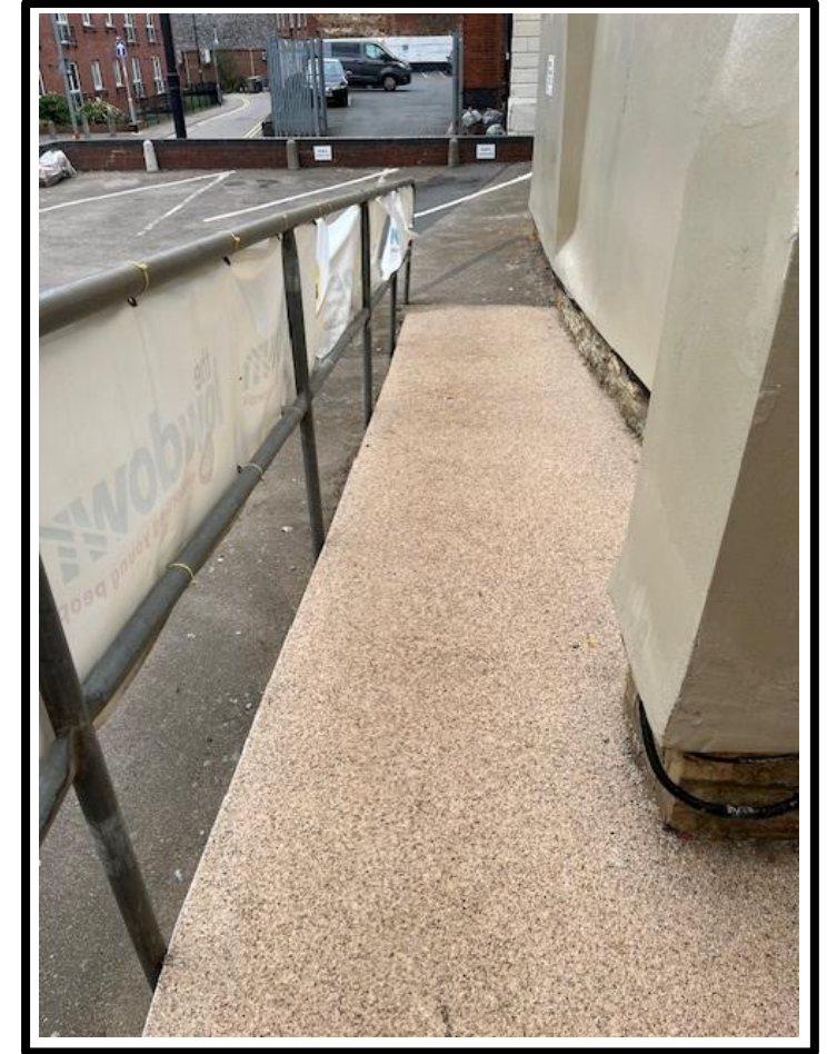
3. Automatic door opens outwards onto accessible ramp to car park.
